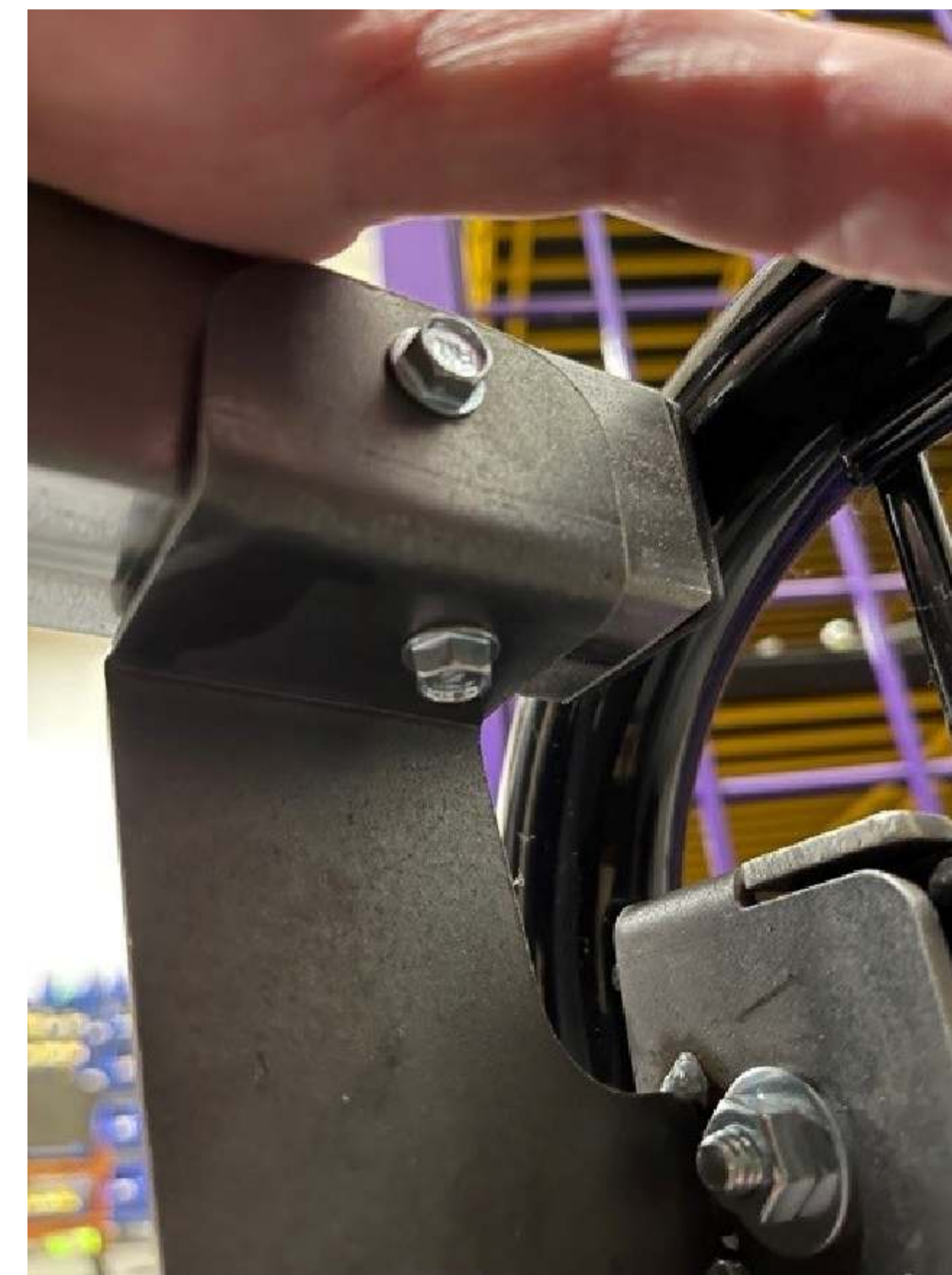
STEP 6: USE PROVIDED SELF TAPPING SCREWS AND INSTALL AS SHOWN ABOVE BOTH SIDES EACH LOCKER OPENING.
