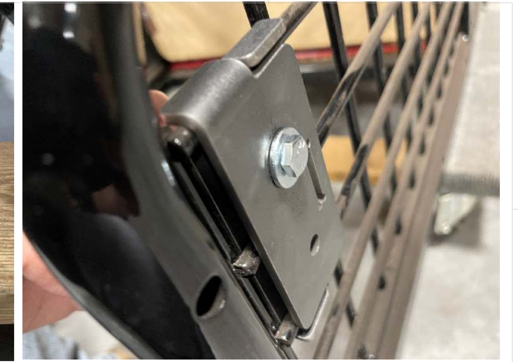
STEP 3: USING HARDWARE SHOWN ABOVE SECURE THE BRACKETS TO EACH SIDE AS SHOWN. REPEAT STEPS 1-3 FOR EACH OPENING.
